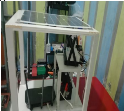
Figure 4 Interface Hardware LBM
