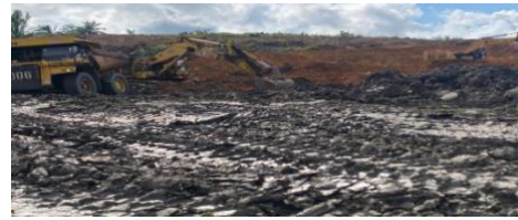
Gambar 3 Kondisi area kerja loading overburde
